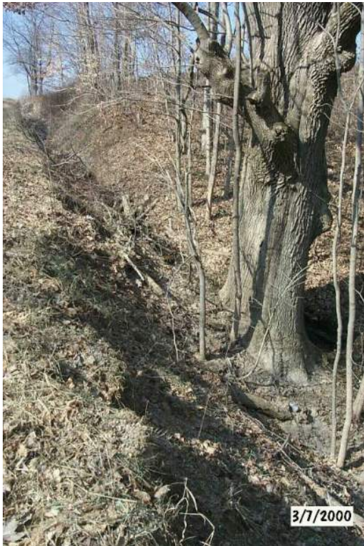
Roadside erosion, Farr Road.
