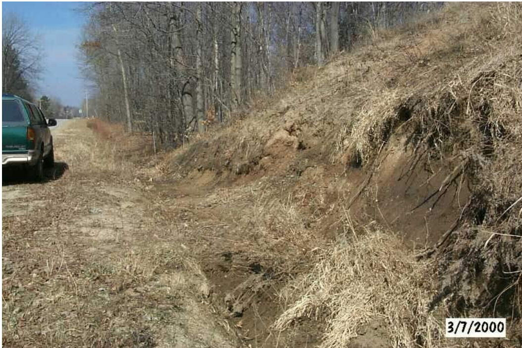
Hilton Park Road near power lines.
