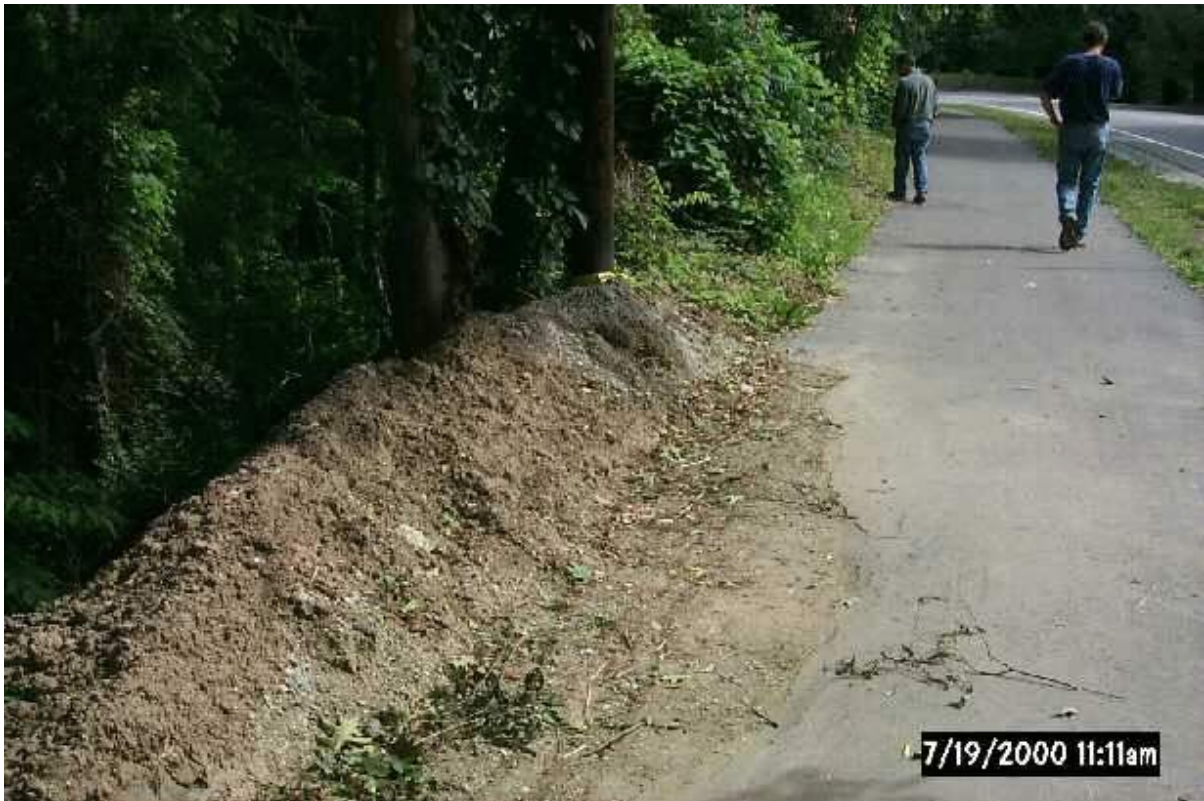
Improper stabilization along paved recreational trail adjacent to Spring Lake.
