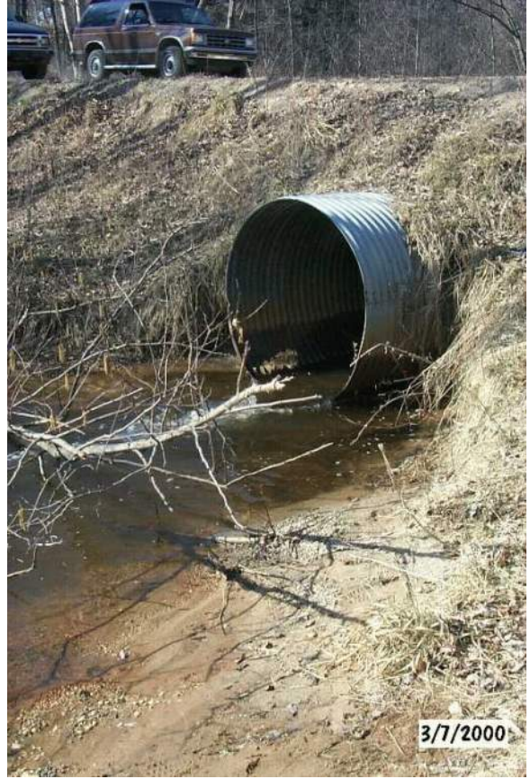
Mt. Garfield Road crossing.
