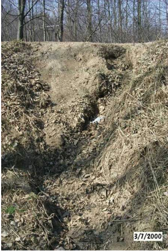
Mt. Garfield Road crossing.
